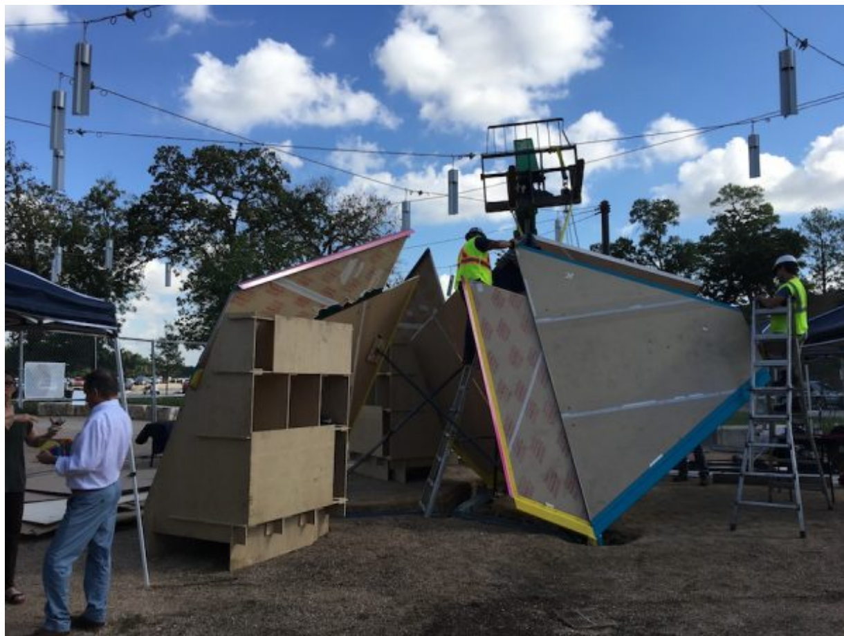
'Mobius Houston' under construction on Sept. 26, 2019.
